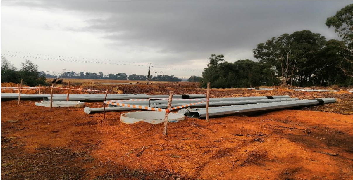
Figure 3: Fitted concrete rings into excavations and placement of steel poles.
