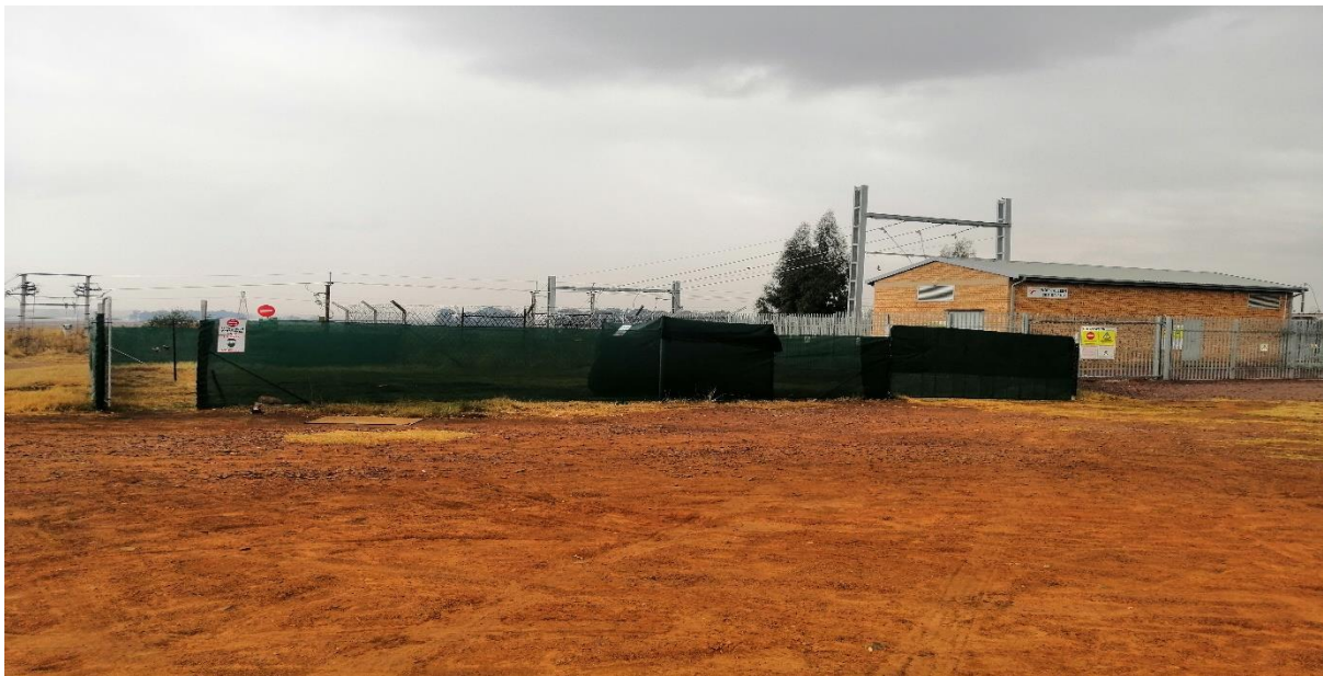
Figure 4: Removal of site office, security guard post and chemical ablution facilities.
